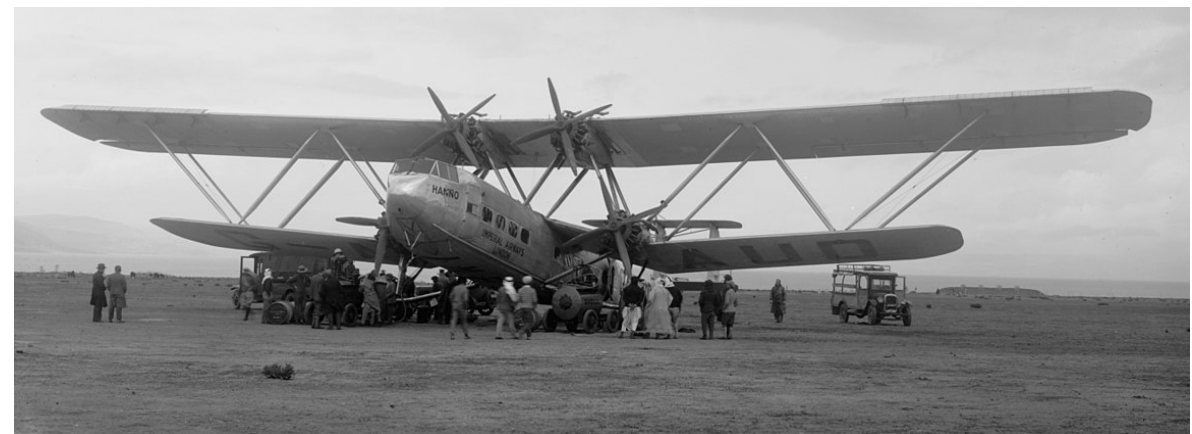
Handley Page HP42 of Imperial Airways (1928) [24pax, 800km, 160km/h, 2000m]
