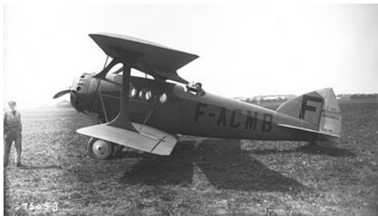
Avion Blériot-SPAD S.33 (1920) [4-5pax, 1000km, 250km/h, 13000m]
